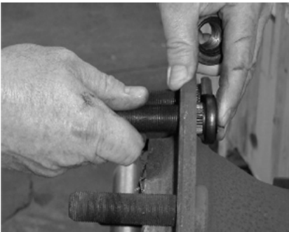
Figure 5: Installing new studs
